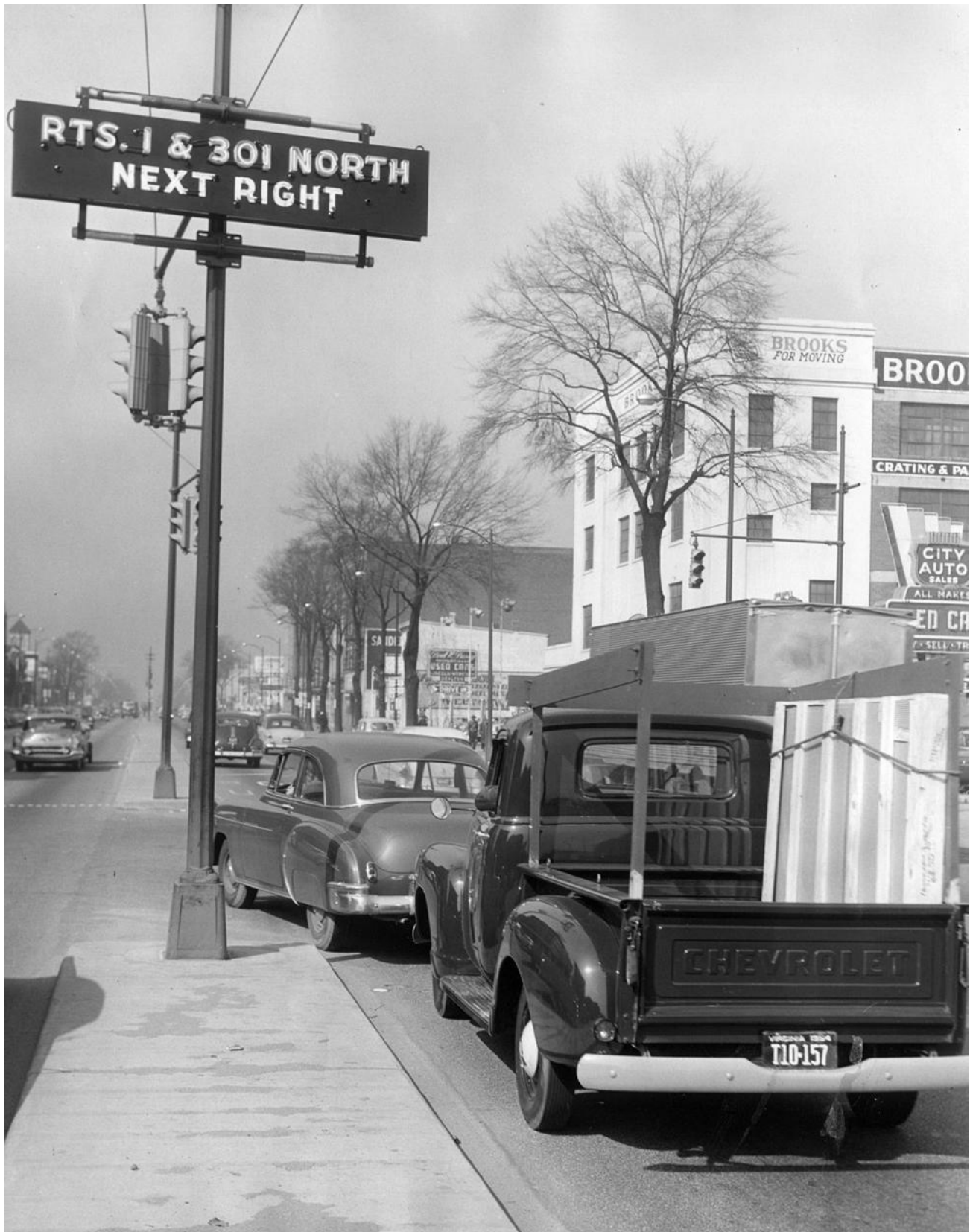
02-22-1955 (cutline): New Motorists' Guide--this large sign recently installed at Ryland and Broad Streets, is designed to prevent accidents and help northbound motorists on U.S. Routes 1 and 201 in Richmond keep on the proper route. The "next right" part of the sign flashes constantly. The Traffic Engineering Bureau said that sign was installed to prevent accidents at Bowe and Broad, where drivers frequently discover they are supposed to turn but are in the wrong lane.
