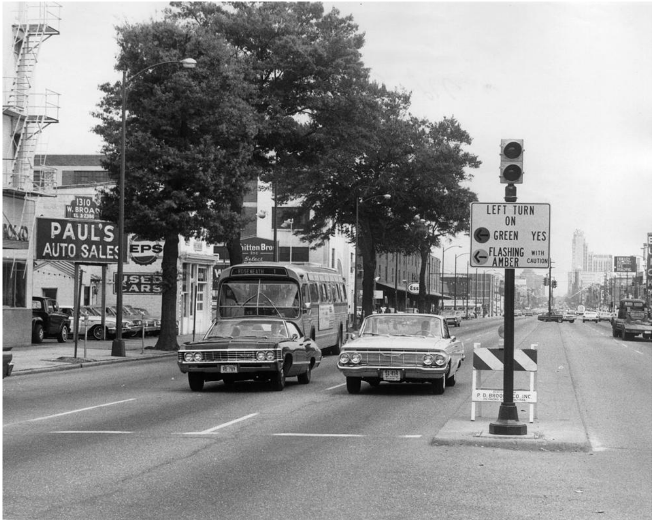
08-15-1967 (cutline): New signal for Left Turns This type of new traffic signal to regulate left turns has been installed at the intersection of Bowe and West Broad Sts. The signal, which faces eastbound traffic on Broad, is designed to give motorists a chance to make left turns without guessing what westbound traffic is doing. If east bound motorists have a flashing green, west boung traffic has a red light. If eastbound motorists have a flashing amber, westbound traffic has a green light and left turns should be made at the motorist's risk.
